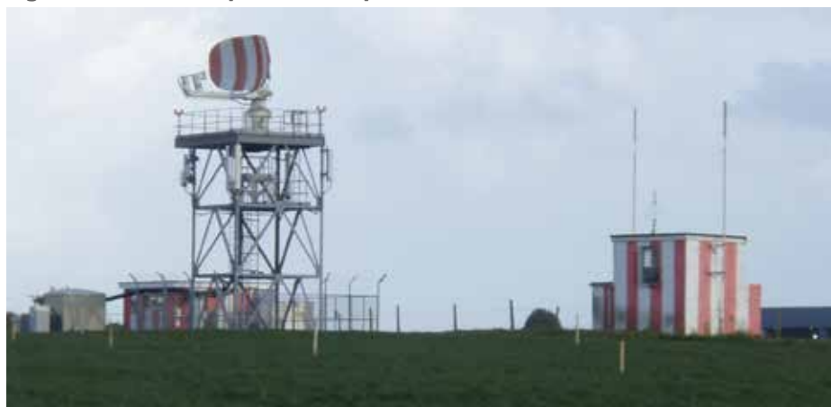
Figure 12.1 — Example of an airport surveillance radar
